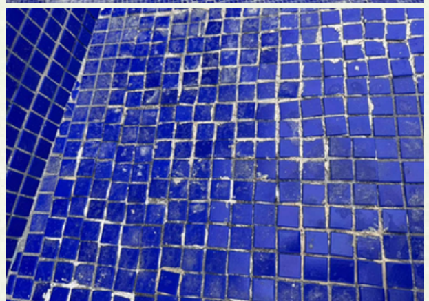
Pool tiles after the repair
